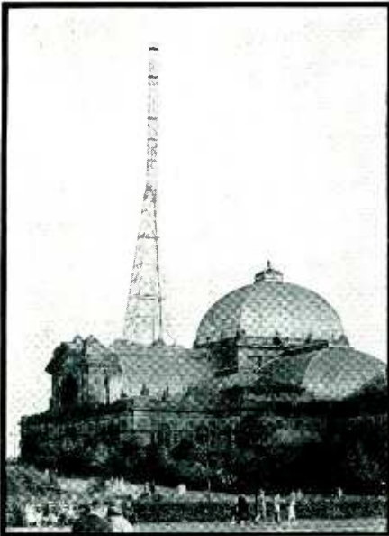
This steel structure, installed on the Alexandra Palace in North London, will radiate sight and sound signals in the forthcoming BBC tests
